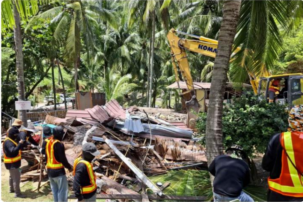
Workers began dismantling illegal bungalows encroaching on Hat Nui in Phuket on Monday.
